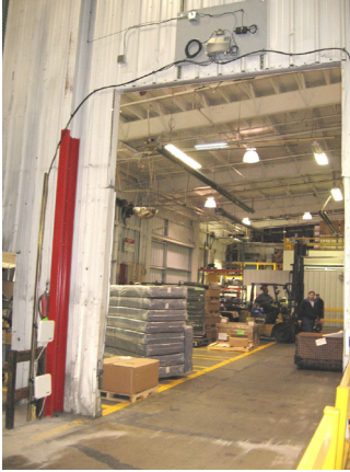
By tagging all totes and tugs and installing Motorola RFID readers and antennas at the doors of the warehouse, in and out movement of parts is automatically tracked and documented.
